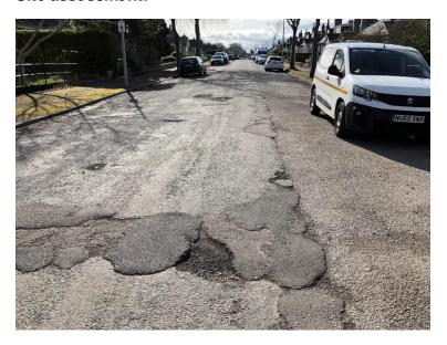
General deterioration in areas of Angusfield Avenue. Multiple utility tracks failing which require remedial works.
