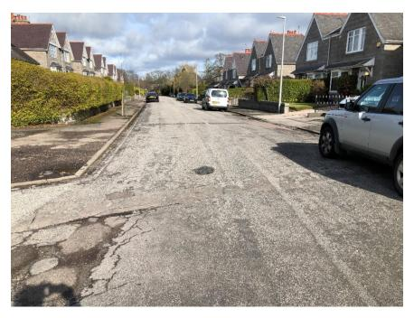
Northburn Avenue is in generally fair condition. Whilst worn, it is free of any significant defects and shows no signs of significant deterioration. The surface appears stable and generally intact. Several localised areas of deterioration present. The road is in good, serviceable condition.
