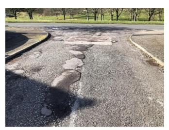
Stronsay Avenue junction with Stronsay Drive; Severe deterioration with multiple repairs.
