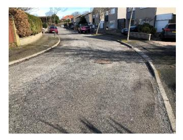
General condition of Stronsay Avenue. Significantly worn, but serviceable and largely free of major defects. The surface is typical of streets of this age. The condition does not present danger to road users and is unlikely to suffer significant and rapid failure.
